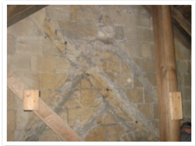
Roof lines (raggles) showing different building phases from inside the loft
